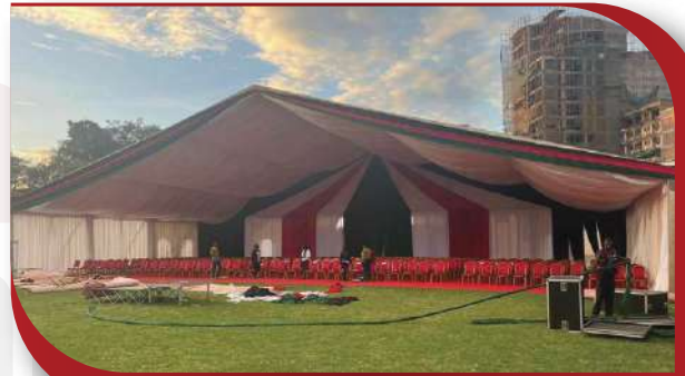
A - Frame Tent Under Construction (Before the event)
