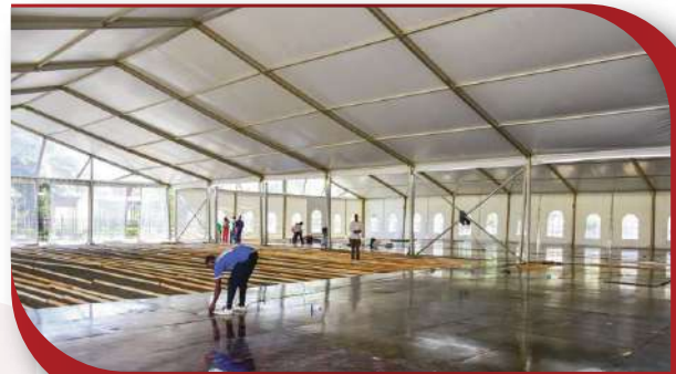
A - Frame Tent (Flooring Construction)
